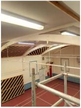
The main roof structure is a series of king post, curved collar-beam trusses with wall-posts on corbels. Each truss has an eaves-level horizontal metal tie-bar with vertical steel hangers from the curved collar beam – see photograph on the left. The trusses support purlins which in turn support rafters. It is likely that the shallow curve of the collar-beam necessitates the horizontal metal tie-bar. All the visible trusses, apart from
