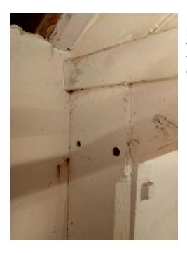
It is not clear why all but one of the tie-bars has been replaced and set at a slightly higher level. In the photograph opposite, the pair of holes below the horizontal steel bracket are we believe the original tie-bar bracket bolt-holes.
