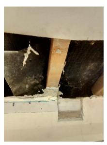
An opening was cut in the plasterboard to inspect the roof timbers at eaves level at a point mid-way along the gymnasium on the west elevation. All timbers appeared to be in good condition with rafters at that location from sawn timber that is probably less than 20 years old. See photograph opposite.
