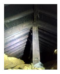
We gained access to the high-level hatch above the gymnasium floor and were satisfied that the roof timbers which were visible from that location are in good condition. See photograph opposite. It was not possible to gain access further into the roof space beyond standing in the hatch-opening. This was due to lack of head-space and excessive amounts of mineral wool at the opening.
