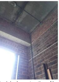
reflective cracking resulting from a joint between recent and original construction. No further action required except to repair the render band incorporating a movement joint.
