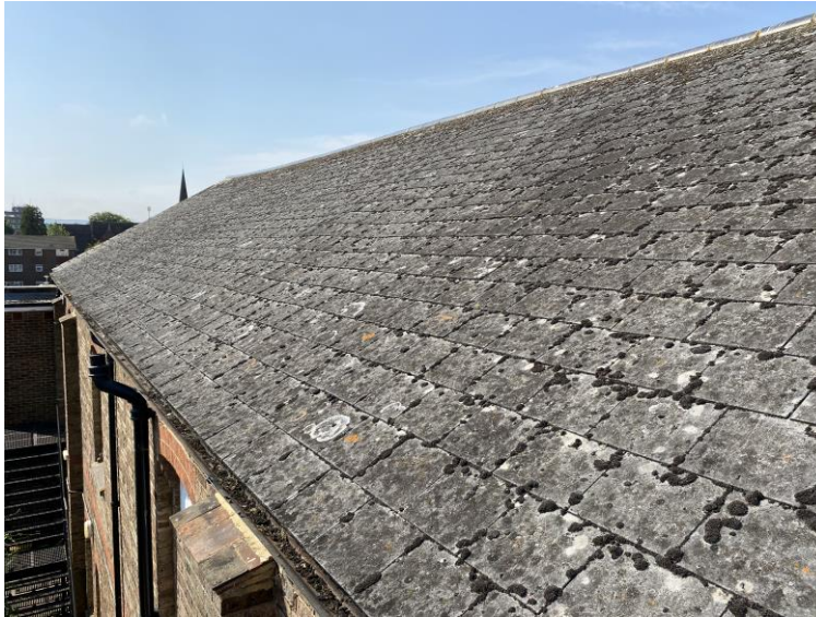
Undulations to east roof pitch.
