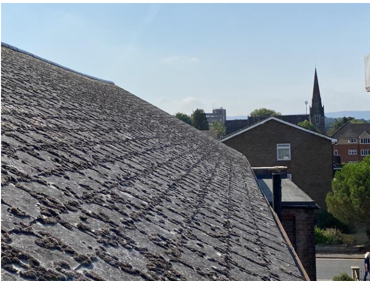
Undulations to west roof pitch.
