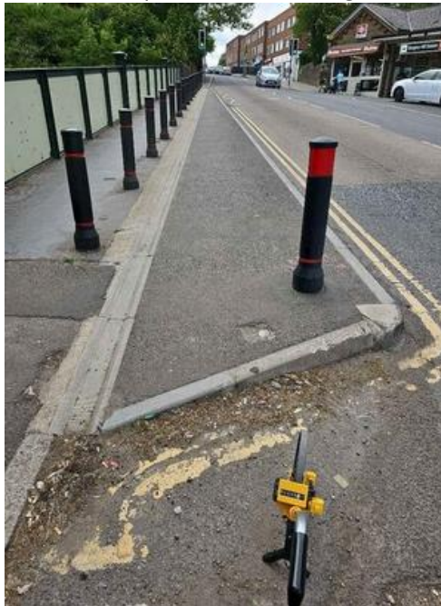
Evidence of quadrant kerb being struck.
