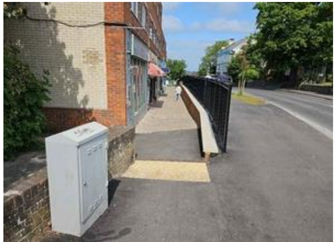
Steep gradient where footpath and foot/cycleway join.
