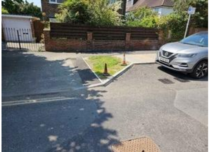
High spot within new asphalt
