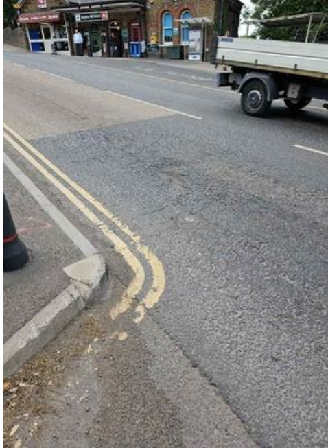
Evidence of quadrant kerb being struck.
